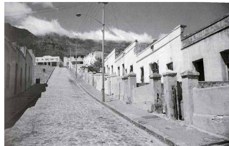
Fig. 2.15. Hosrtley Street Historic Image
